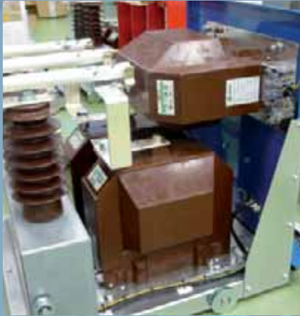
› UCL-7 Voltage transformer compartment in medium voltage switchgear.
