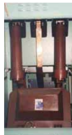
> Support type voltage transformers with fuse VCT type.
